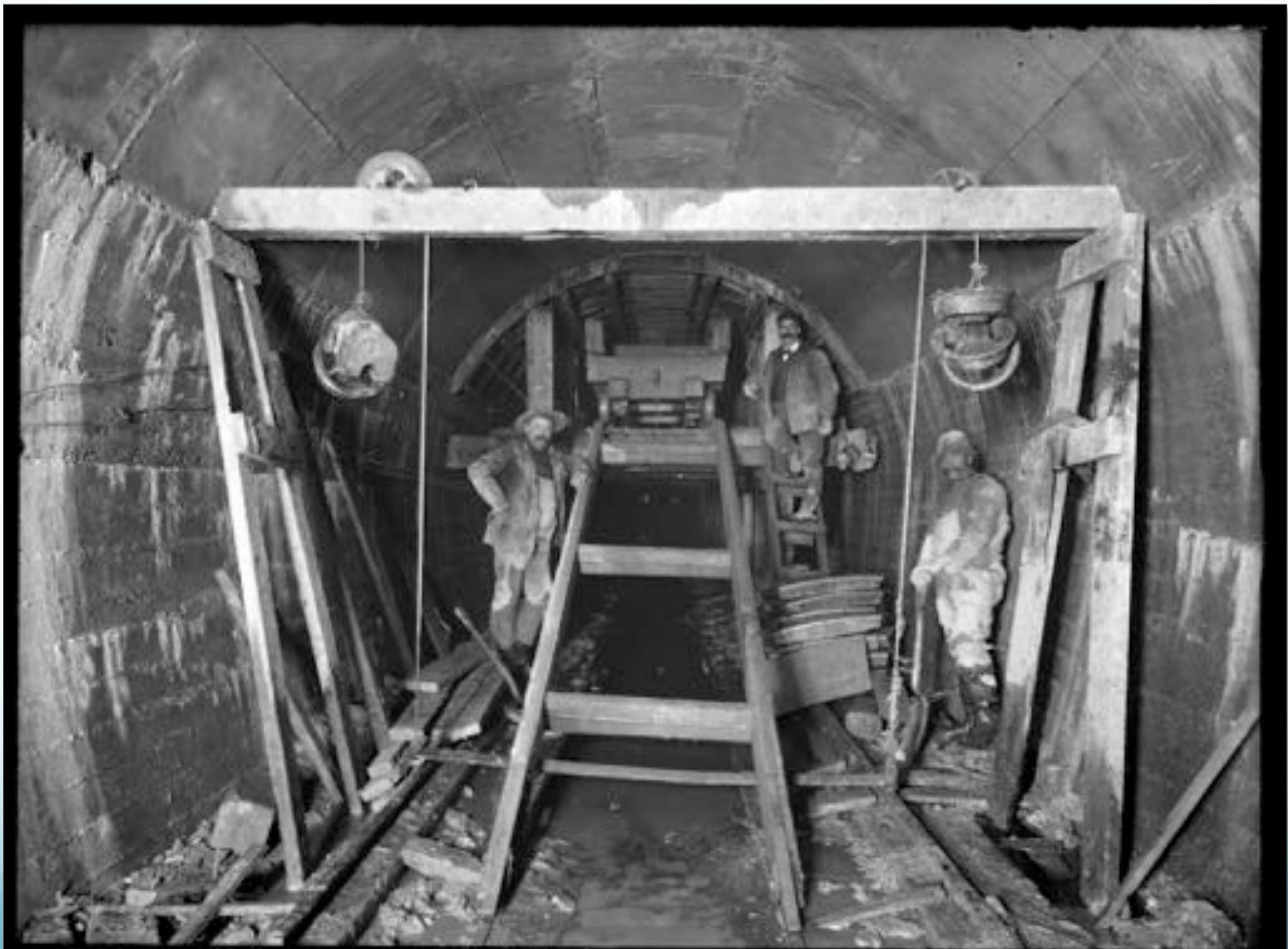
WESTON AG.SEC.13. TRAVELER FOR ARCH WORK IN TUNNEL.
