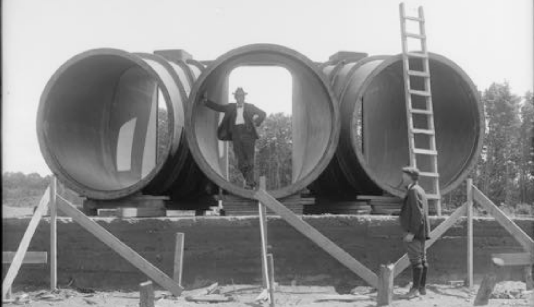
WESTON AG. SEC. 6 CASTINGS AT SIPHON CHAMBER AUG. 7, 1902
